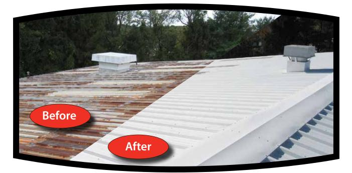
Need to extend the life of your metal roof? Firestone Building Products Fluid Applied Metal Roofing Systems will restore your metal roof and improve building performance while saving you money. The Firestone elastomeric roof coatings are formulated with a 100% acrylic polymer that provides outstanding adhesion, excellent water protection and superior durability.
